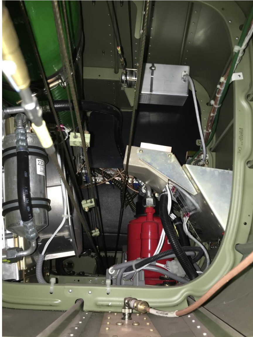
Figure 8 - Visually Inspect from Access Panel
